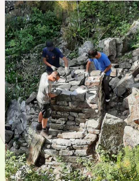
Consolidation of the base of the ironworks' supply canal (2024)
