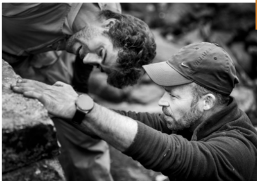
The conservation works of the Madriu forge (2021-2024)
